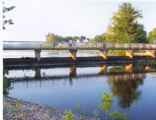
Milford Pond Dam
